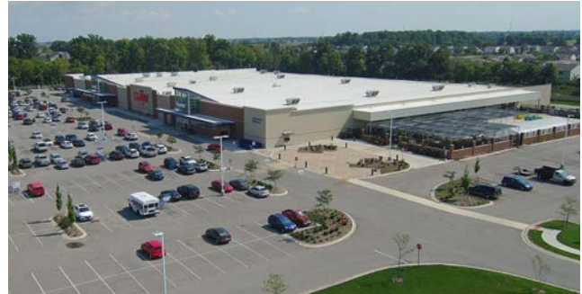
Meijer in McCordsville continues to draw regional shoppers.
