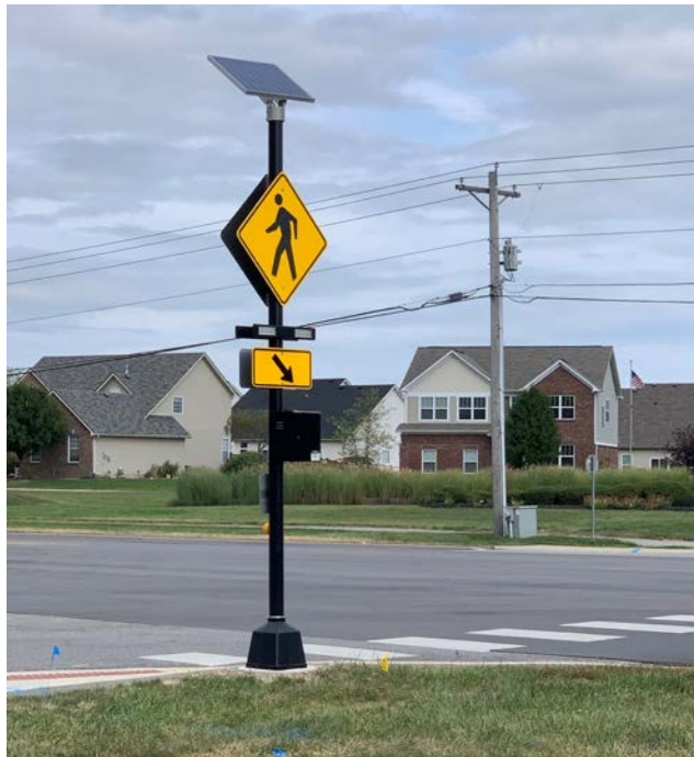
The Town recently installed pedestrian crossing signals at three crossings on CR 600 West.
